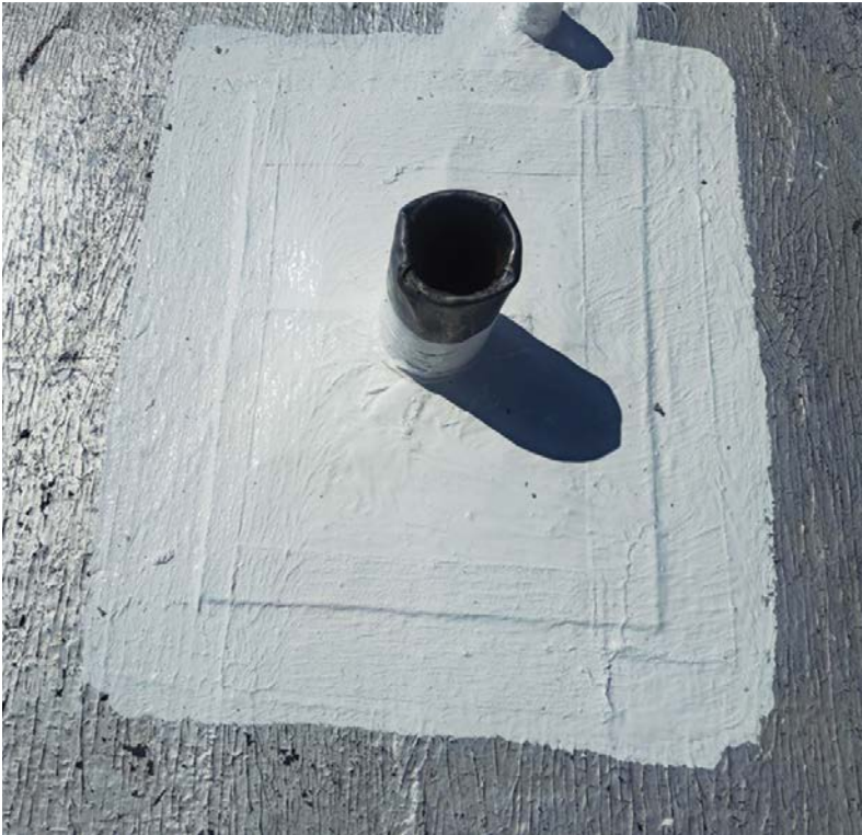
Hybrid flashing-grade sealant used to flash a pipe penetration on a previously aluminum-coated roof.
