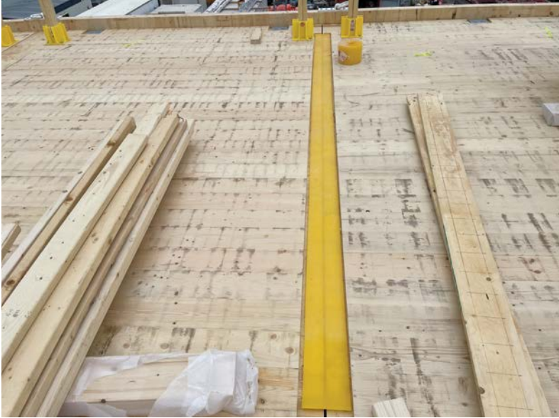
Isolation pad in between and on top of continuous cross-laminated timber (CLT) panels. PHOTO COURTESY AERCOUSTICS ENGINEERING LIMITED
