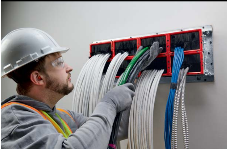
Example of firestopping using cable pathway devices.
