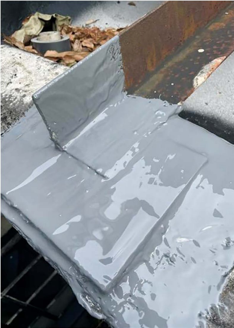
Hybrid flashing-grade sealant used to flash an irregular roof detail. PHOTO COURTESY BITEC INC.
