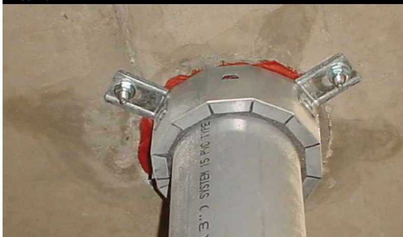
Example of intumescent firestop collar for combustible pipe firestopping.
