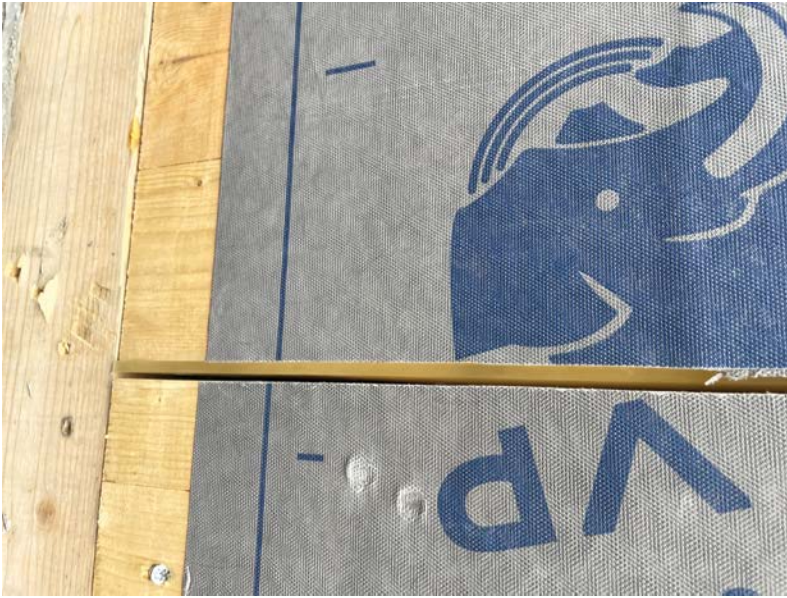
Vertical junction gap between continuous cross-laminated timber (CLT) panels.
