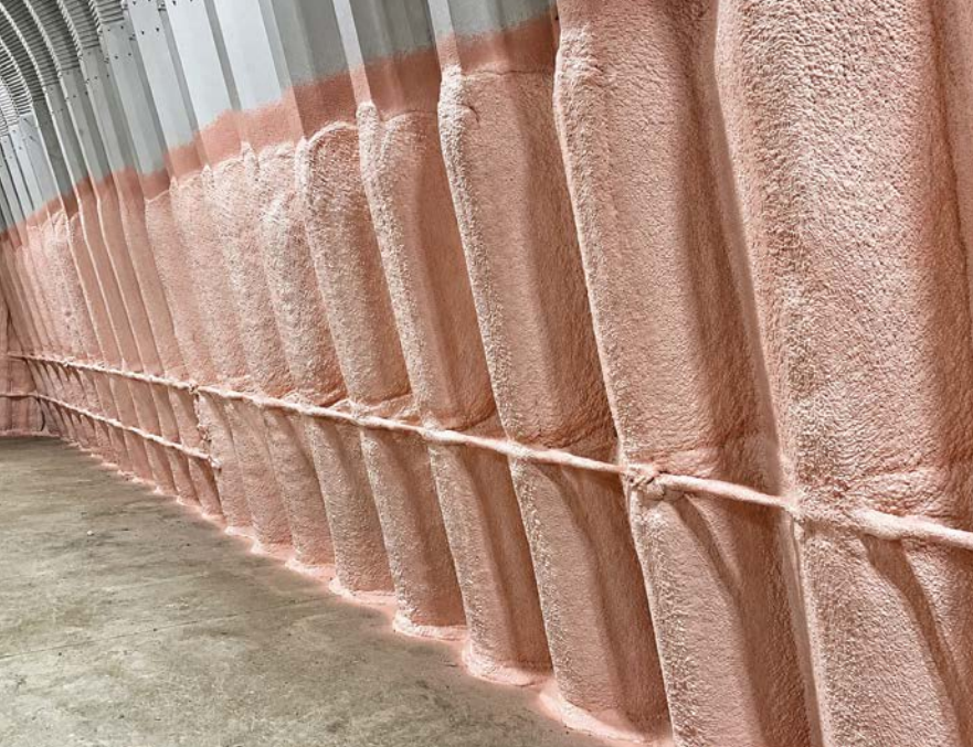
Closed-cell spray foam installed within a curved steel assembly, demonstrating the material's ability to conform to irregular geometries while maintaining all control layers.
