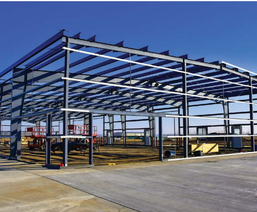
Many metal building systems are particularly well-suited to industrialized construction.
