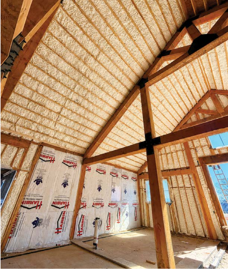
Open-cell spray foam applied along the underside of a cathedral roof assembly.
