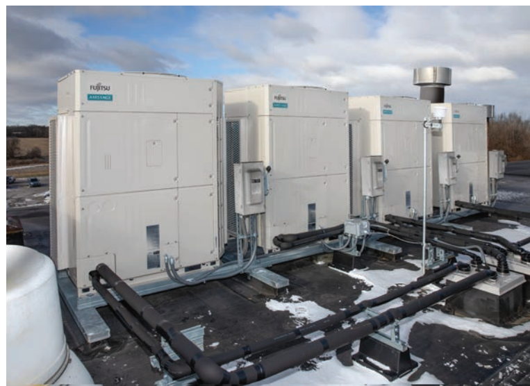
In some light commercial applications, the best solution may be to install several multi-zone mini-split heat pumps.
