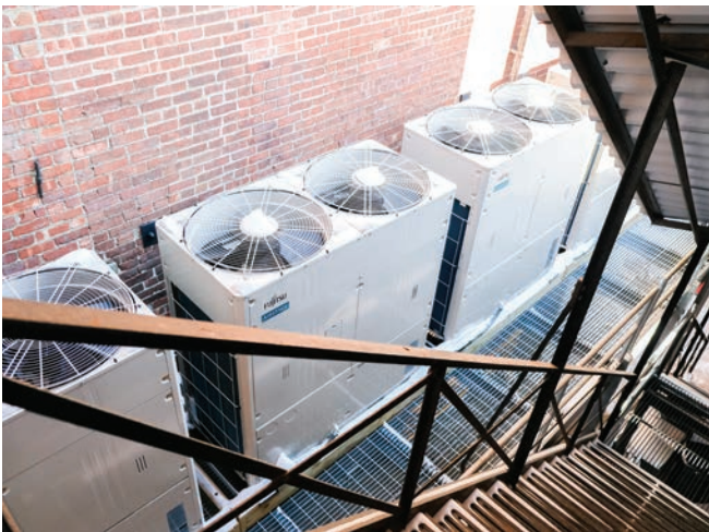
Modularity and design flexibility are some of the advantages of heat pumps, especially in retrofit applications.
