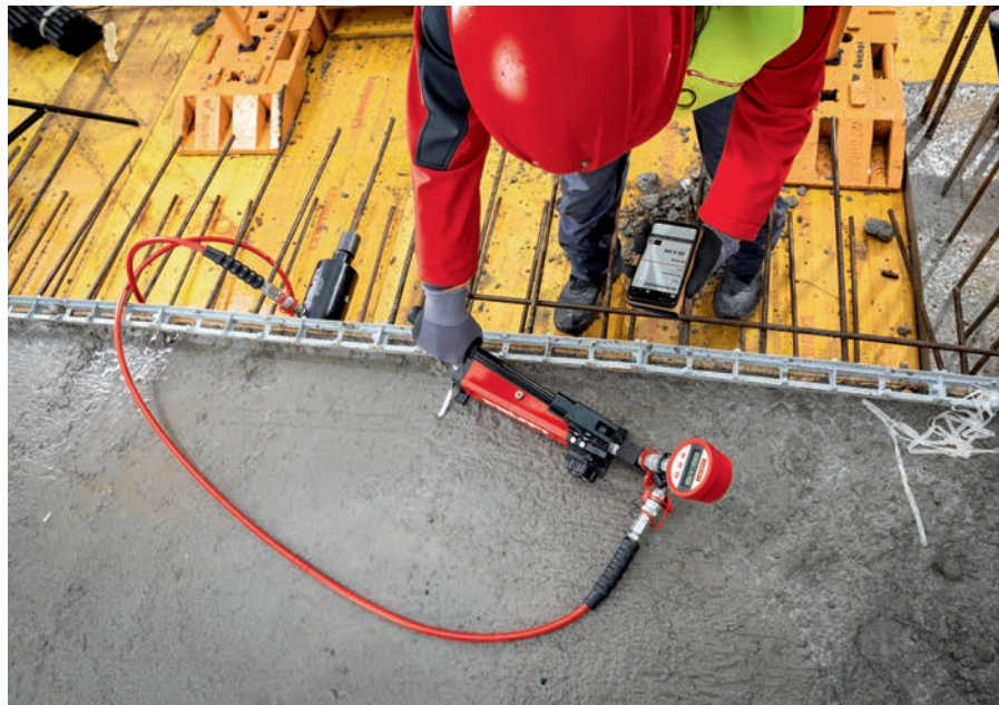
On-site post-installed rebar pull test on concrete.
