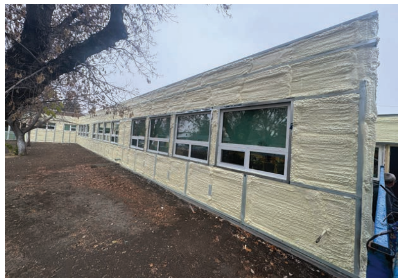
The four control layers are essential to resilient and durable building enclosure design. Vapour-permeable insulation materials can allow assemblies to dry when required by allowing vapour to diffuse through the wall system.
