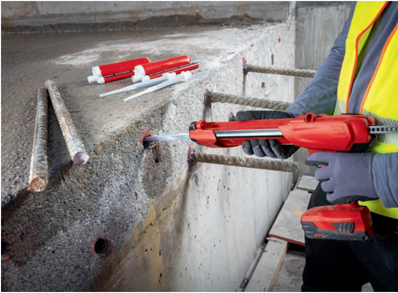
Post-installed reinforcing bar installation using an adhesive anchoring system.
