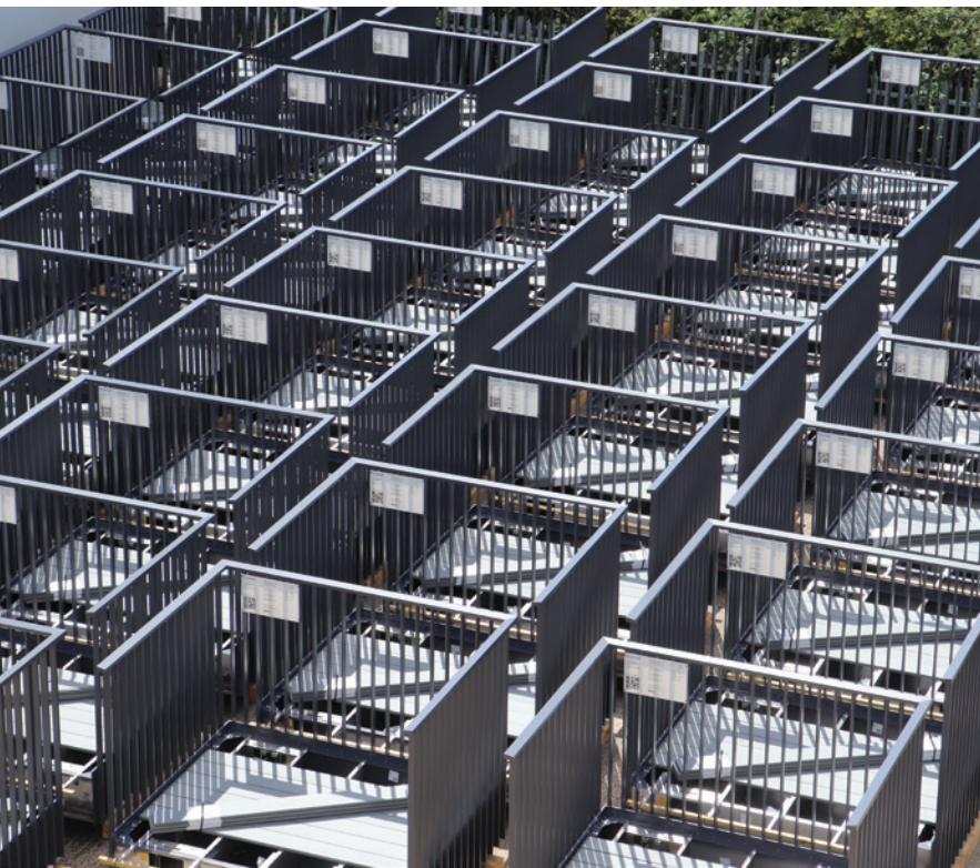
Factory-built balcony assemblies illustrate the efficiencies of modular construction, including improved quality control and reduced on-site labour. Performance ultimately depends on how well systems accommodate site tolerances and interfaces.
