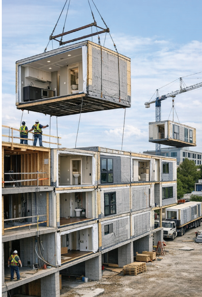
On-site assembly of modular units.
