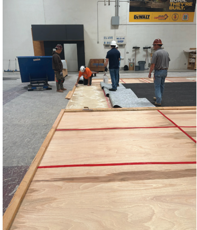
Sports flooring systems are highly specialized assemblies, requiring certified installers to meet warranty requirements and ensure precise performance.
