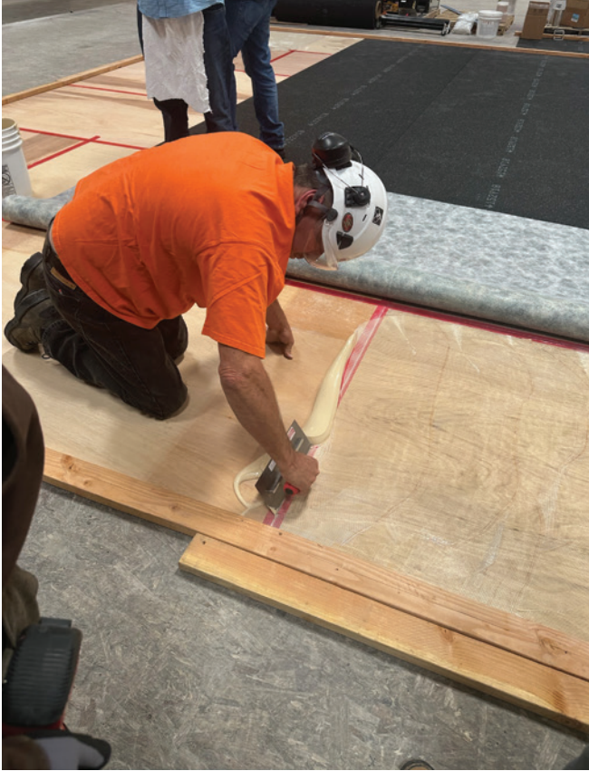
Meeting performance metrics depends on precise substrate preparation and pad installation.
