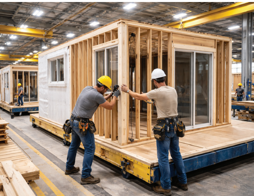
Workers constructing a modular unit off-site in a factory setting.
