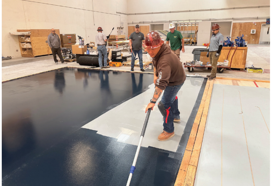
Pad-and-pour polyurethane flooring is a seamless, poured-in-place system made of a resilient pad layer installed over a substrate and finished with a liquid-applied polyurethane topcoat.
