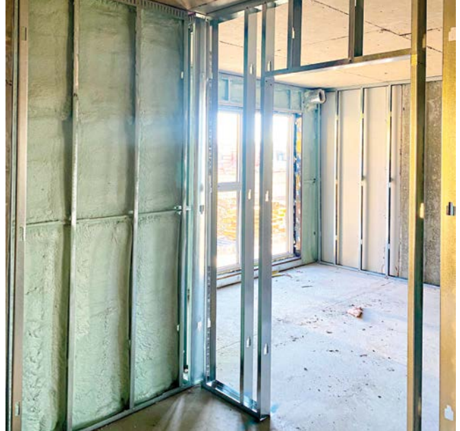
Steel framing and sprayfoam combine to support long-term thermal performance.
