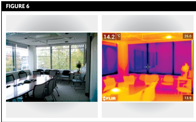
Visual and infrared images illustrating enclosure-driven surface temperature variation in a perimeter space.
