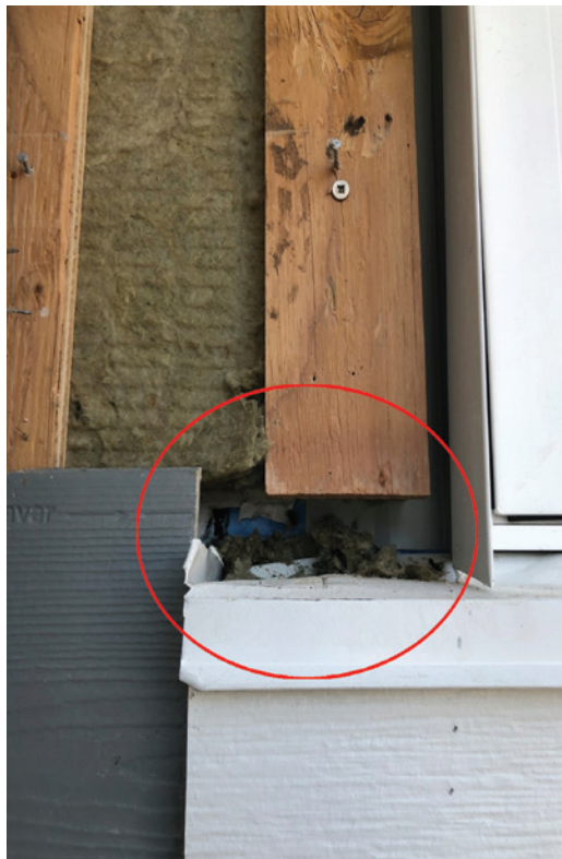
Compromised insulation, damaged by rodents, found within the cladding sections near the window jamb and head.
