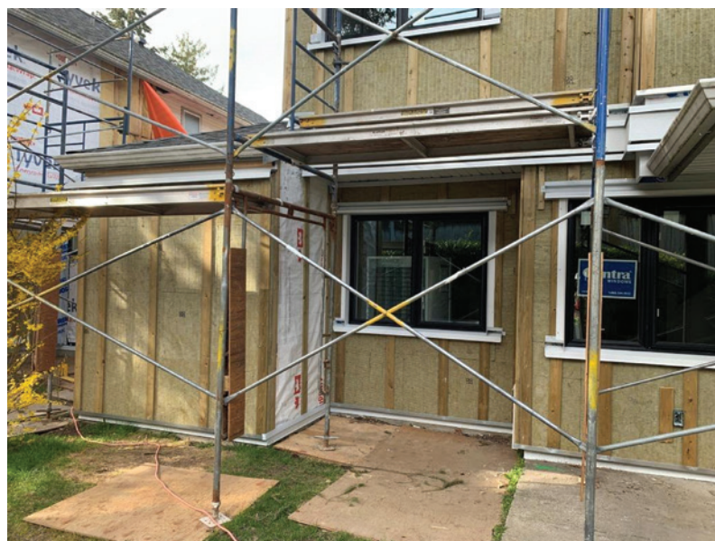
Demonstrates the proper installation of insect screens around pressure-treated strapping and exterior insulation.
