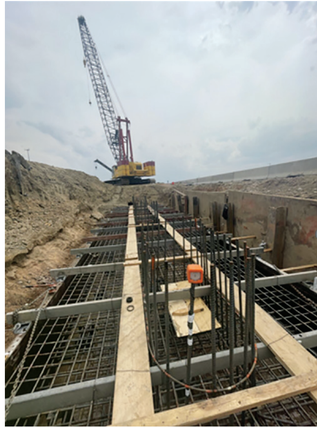
Footings are typical mass concrete structures that require concrete monitoring to ensure compliance with thermal control plans.
