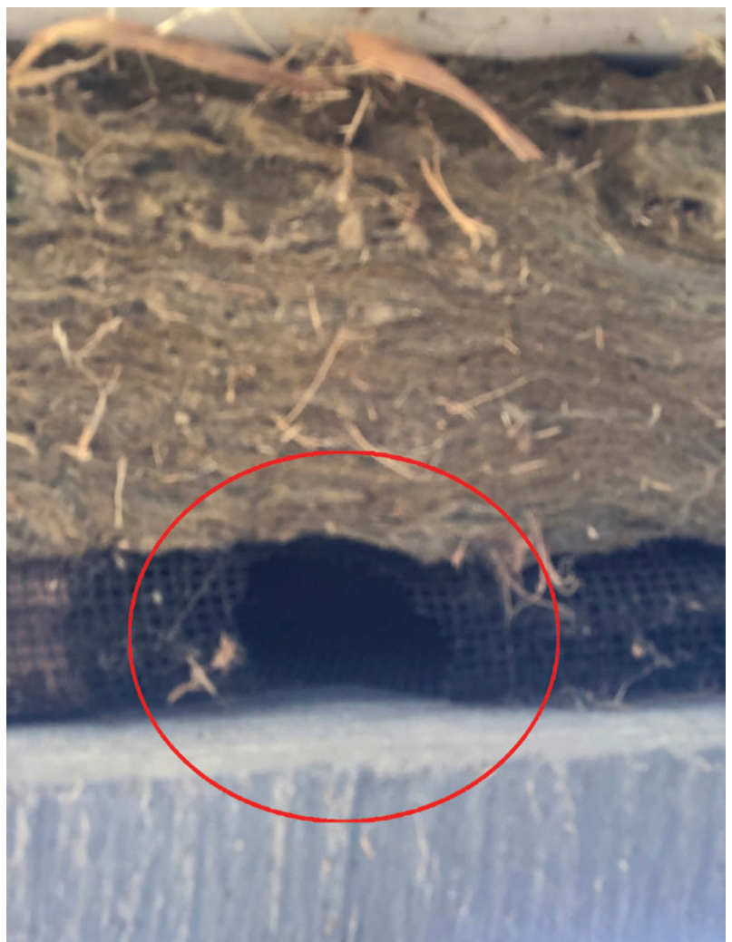
Rodent-induced breaches in the insect screen, allowing rodents to establish nests within the wall cavity. The fibreglass insect screen proved insufficient in terms of durability and strength.
