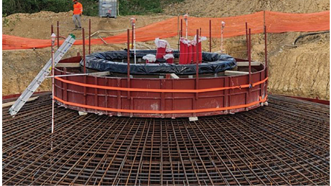
Reinforced wind turbine foundation before mass concrete pour at Punta Lima Wind Farm, Naguabo in Puerto Rico.
