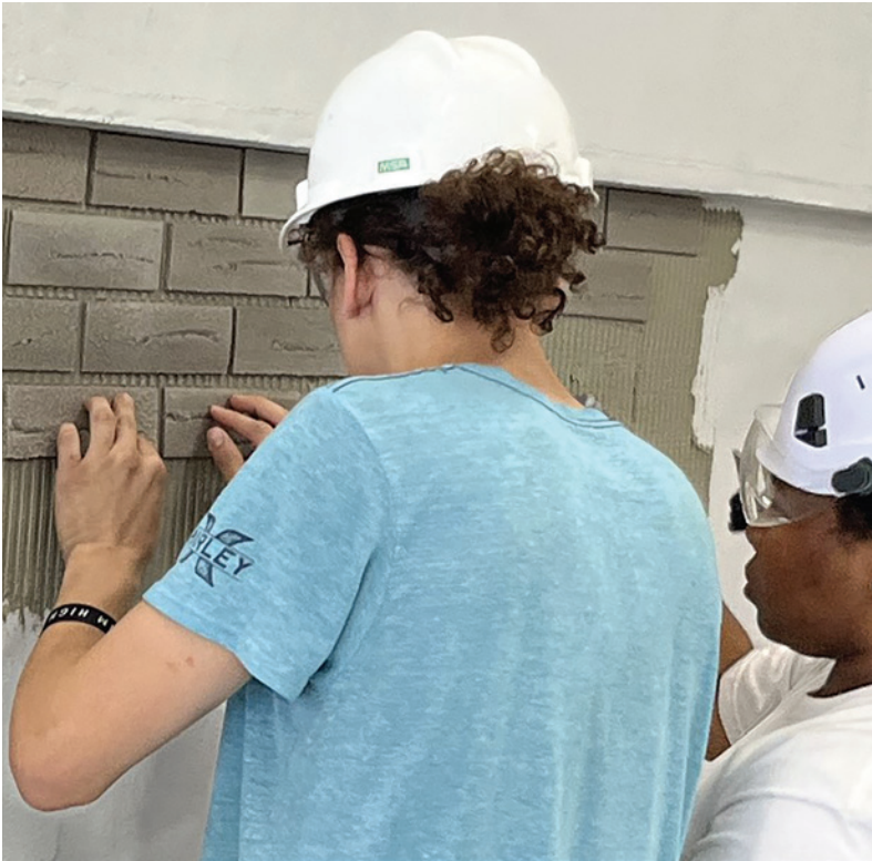
Field application showing brick panelling, joint layout, and colour range—an essential step for visual approval and quality control.
