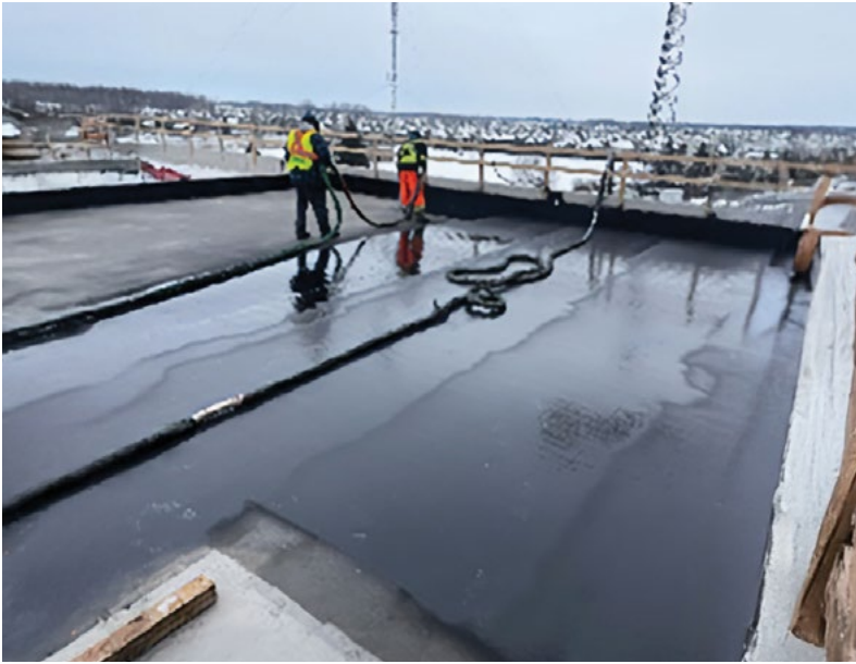
Podium deck application.
