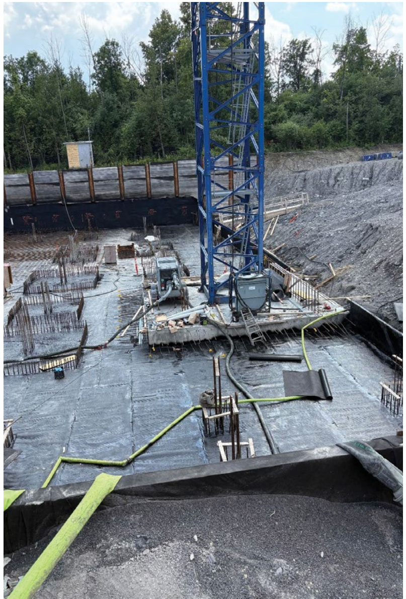
Bathtub waterproofing application.
