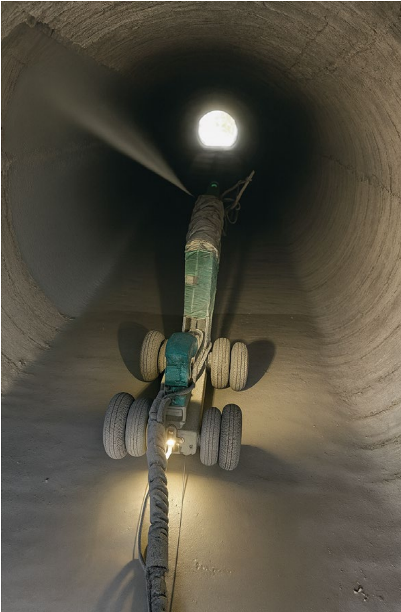
Sewer lining with polyurea using robotic arm.
