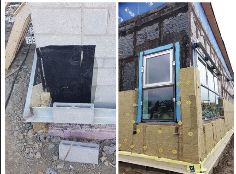
Knife plate standoff on a concrete block brick veneer wall assembly in a school.
