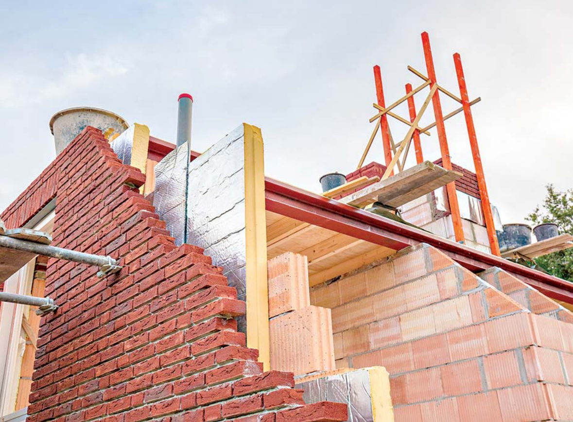
Cavity wall construction in progress: insulation panels placed between brick and block layers help reduce heat loss, manage moisture, and improve overall building efficiency.
