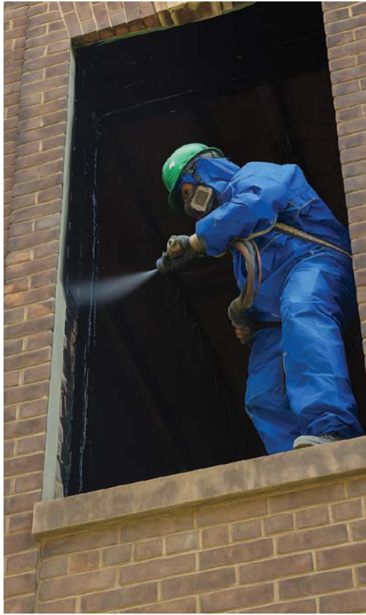
Polyurea being applied to a window opening to tie in an air barrier system.
