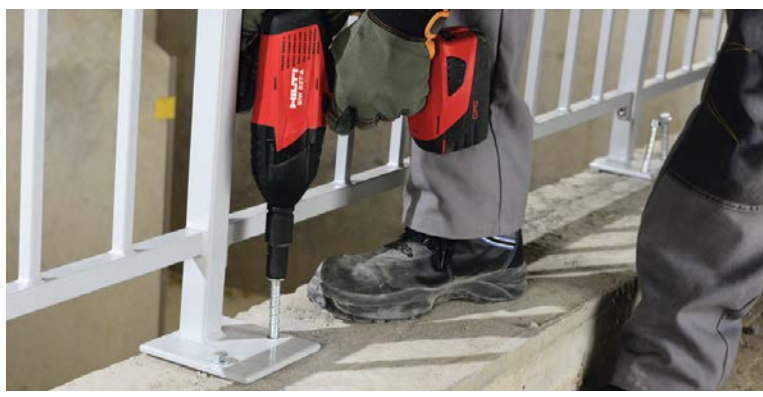
Post-installed screw anchor installation.
