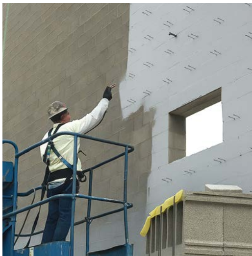
A liquid-applied air barrier forms a seamless membrane directly on the substrate, simplifying detailing around penetrations and transitions.
