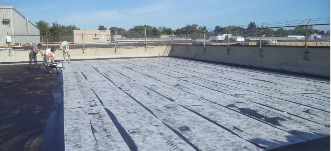
Installation of first ply and reinforcing for hot-rubberized waterproofing system.
