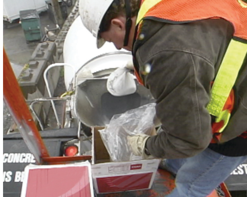
Crystalline waterproofing in water soluble bags is added to the back of a ready mix truck.
