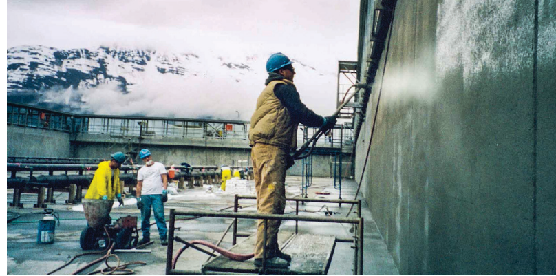
A protective layer of crystalline waterproofing is applied to the Valdez Marine Terminal water purifying tanks in Prince William Sound, Alaska.
