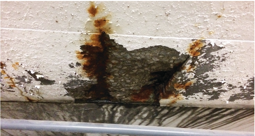
Deterioration as a result of waterproofing failures.
