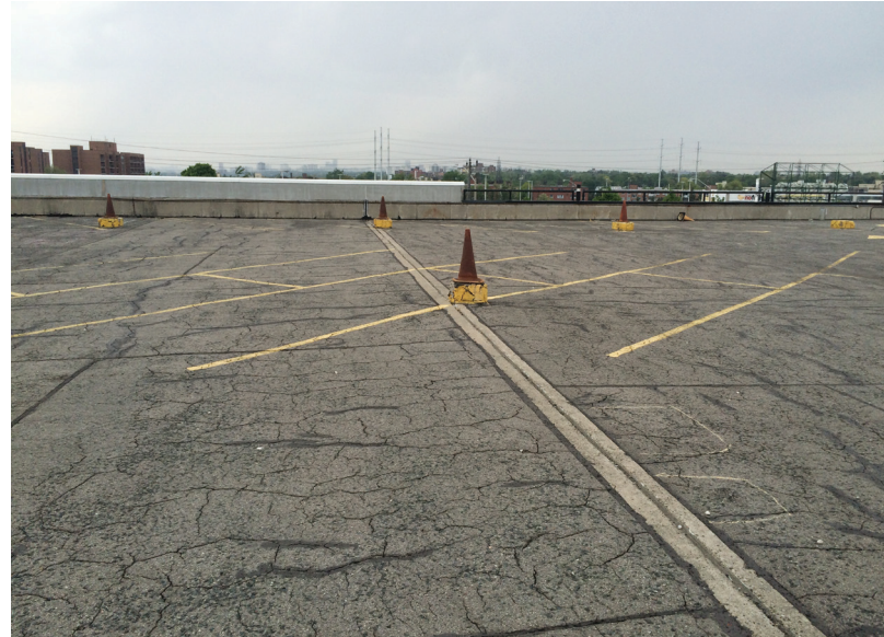
An example of deterioration of a thick waterproofing system on a roof deck.
