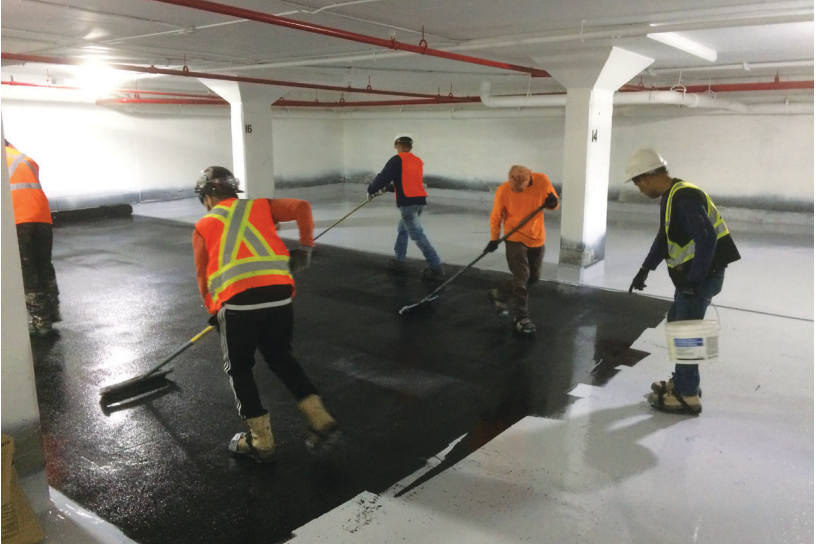
Wearing surface application for a thin traffic deck coating system.
