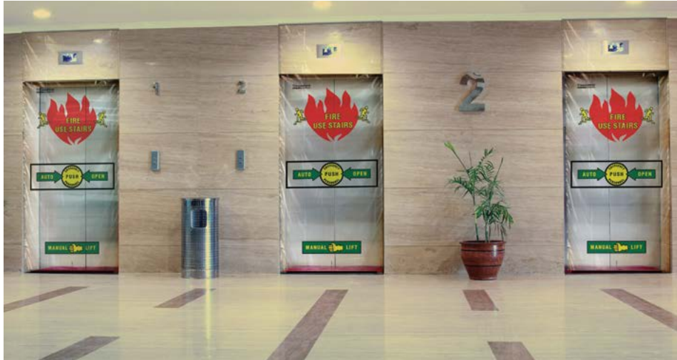
Elevator smoke containment doors seal off hoistway openings from vertical smoke migration.
